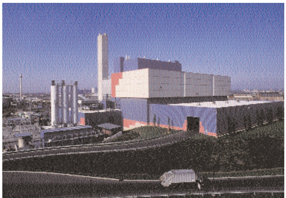
An Efw facility in Essex, New Jersey, US. PHOTO: AMERICAN REF-FUEL
