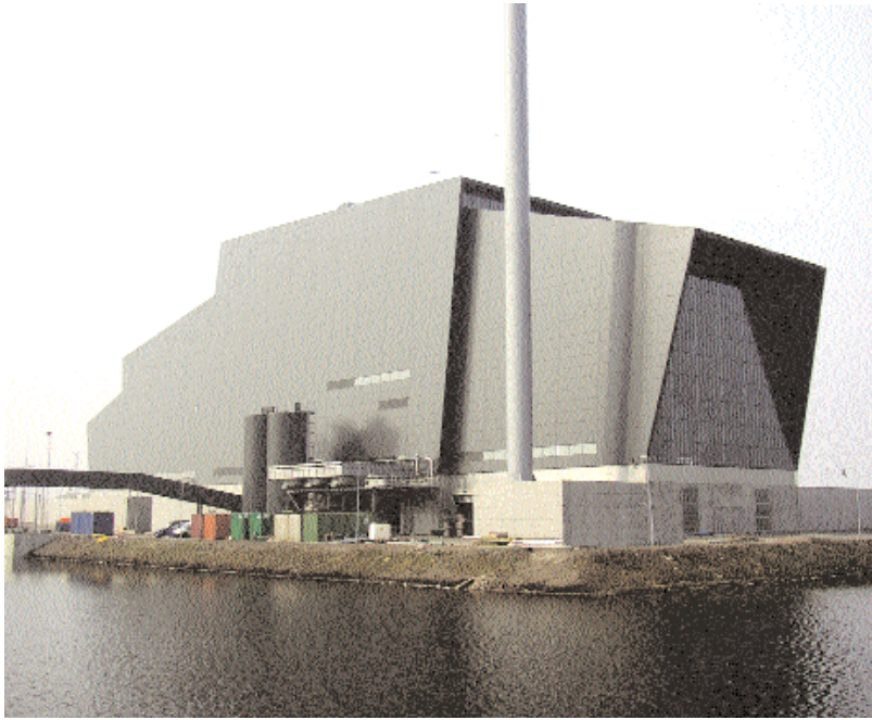
Incinerator plant in Denmark: the disposal of MSW represents a chance to recover the energy available in it. PHOTO: BABCOCK & WILCOX VØLUND APS
